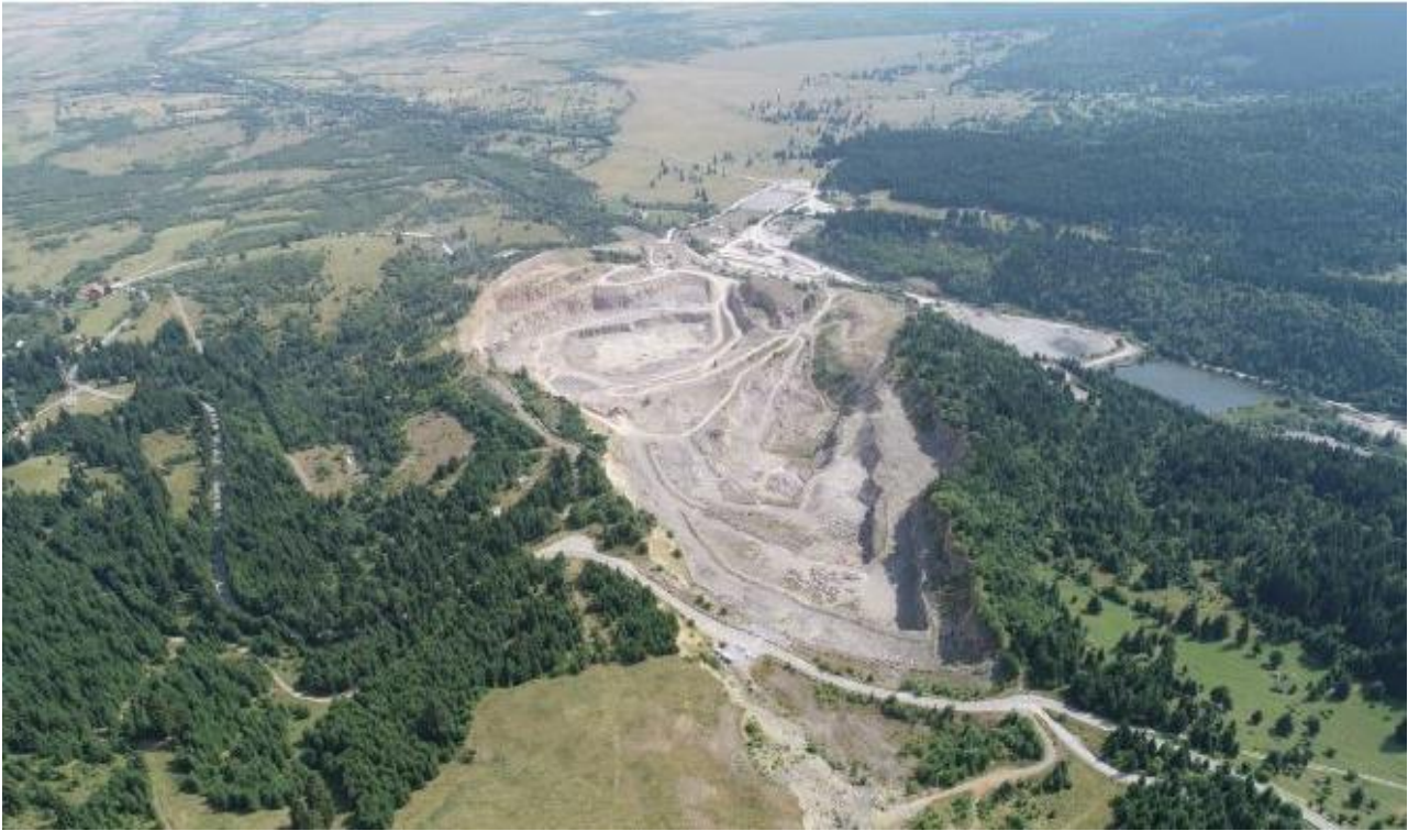
Fig. 1. Upper view of Suseni quarry (from the tender)
